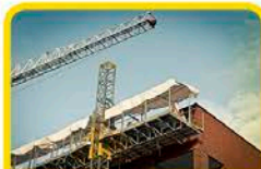
Tower cranes and hoists
